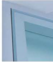
Glazed to wall abutment
