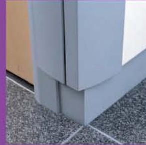
90 degree corner doorset to solid
